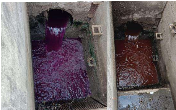
Picture 4-8: Dyeing waste is received at 7 MLD STP inlet chamber
